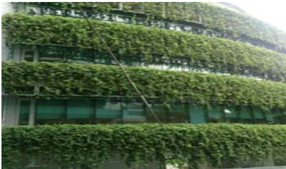
Figure 4. Example of Wall-Climbing green wall at Li Ka Shing University, Singapore
